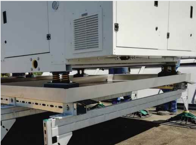
Unit installation in the drip tray
