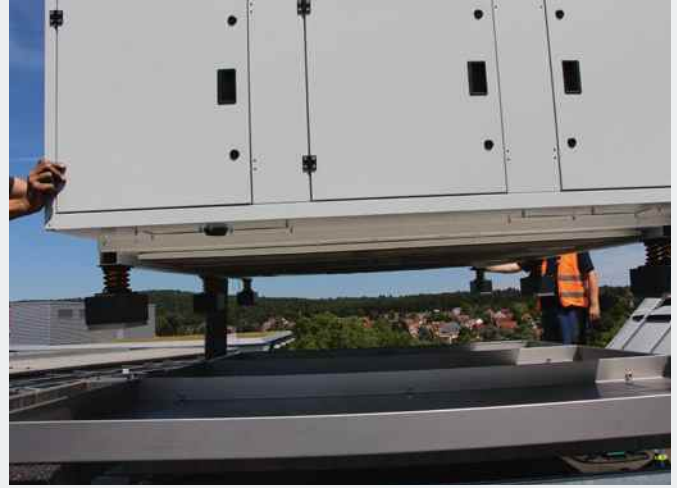
Unit installation with pre-mounted Isotop DT
