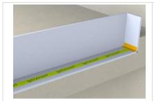
7) Seal joints and corners with adhesive tape.
