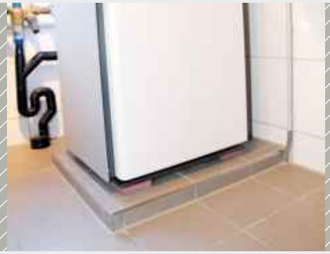
Sylomer® discrete bearings for a heat pump
