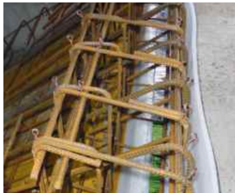
Stair bearing SB10 under in-situ concrete stairs
