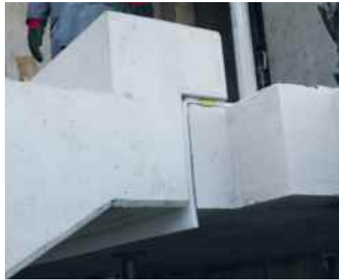
Staircase bearing SB10 under Precast concrete stairs
