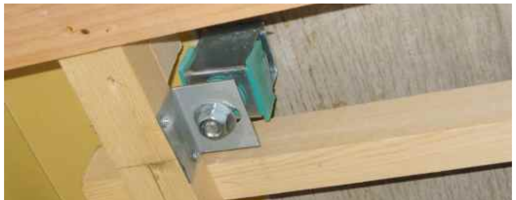
Acoustics sound insulation for ceilings with Sylomer®
