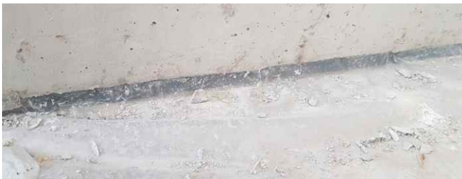
Fig. 3: Slab Track on Getzner high-tech PUR Source: Getzner Werkstoffe
