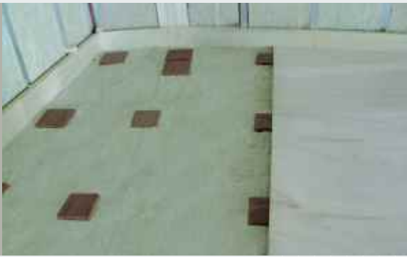
Sylomer® point bearing for vibration isolation of floors
