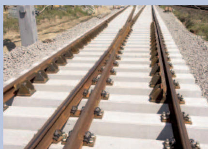
Fig. 1: Turnout with rigid crossing frog and check rails
