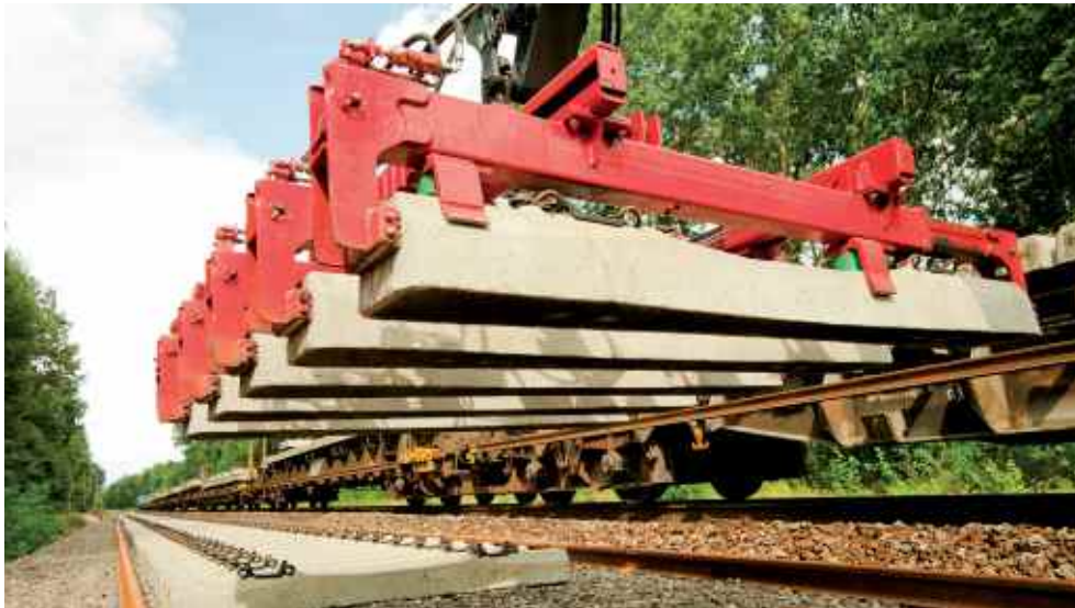
Installation of concrete sleepers fitted with Sylomer pads.
