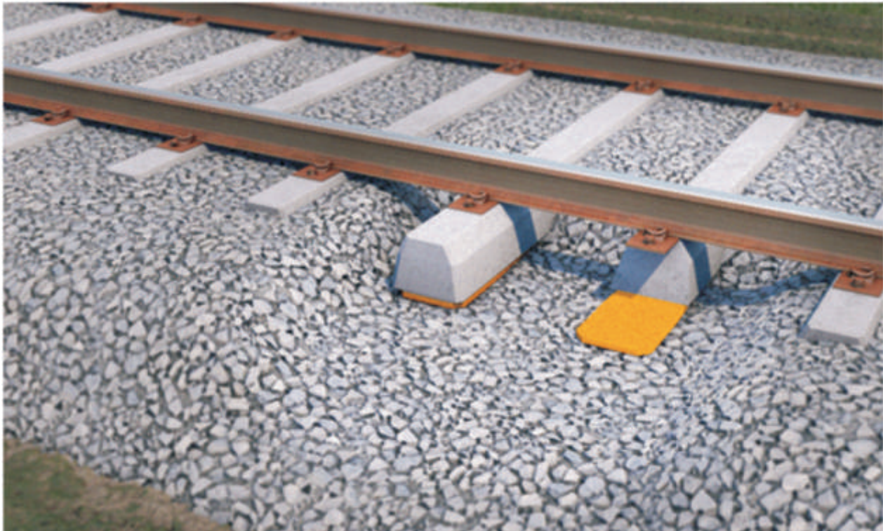
Figure 1: Padded concrete sleepers with polyurethane USP installed in track.
