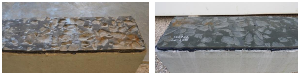
Figure 12: The elastic and plastic material properties of under-sleeper pads combined: forecasted and desired ballast impressions immediately after removal (left) and three weeks later - complete restoration (right)
