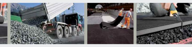
When existing track sections are retrofitted with mats, the laying surface frequently consists of old ballast. In this case, it has proven effective to provide a load distribution layer on both sides of the mat.
