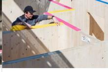
6) Place the elastomers to their final position according to your installation plan. Put the butts bluntly together.
