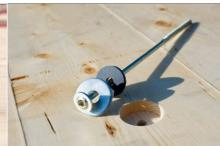
Screw connections need to be pre-drilled. In order to decouple the screw elastic washers are recommended.
