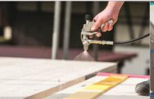
5) Optionally the elastomers can be secured with spray adhesive or mechanically, to prevent slippage during the placement process of the timber elements.
