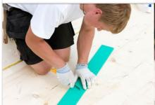
4) Now cut the elastomers to the desired dimensions according to your positioning or installation plan.
