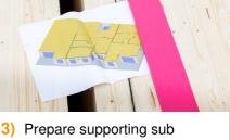
Prepare supporting sub ground according to construction specifications (e.g. sill beam) and mark the position of the elastomers.
