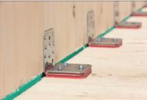
Mechanical connections between decoupled elements need to be equipped with elastomers too.
