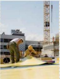
In accordance with the load transfer by the load-bearing walls, Sylomer materials with various rigidities were used.
