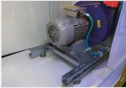
Radial fan in an HVAC system
