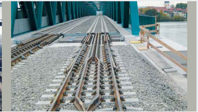
Transition area on a steel bridge
