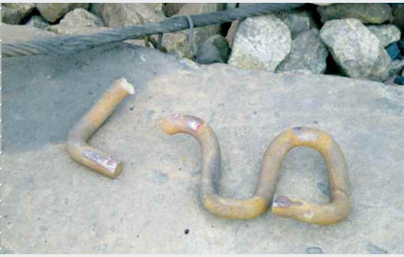
Tension clamp fracture
