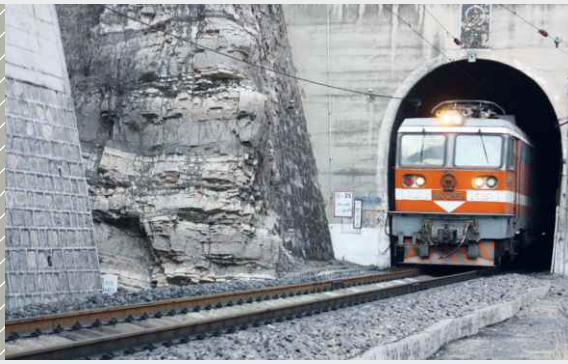
Tunnel on the Fengsha coal line in China
