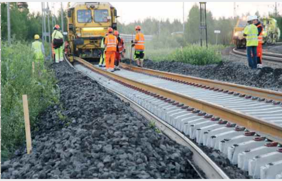
Installation of padded sleepers on the Malmabanan route
