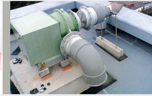
Point bearings for a air handling unit
