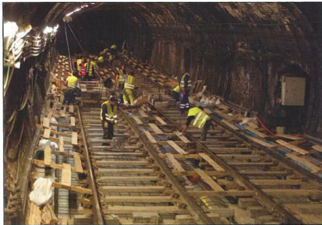
Fig. 7: Final preparations before pouring the initial concrete layer
