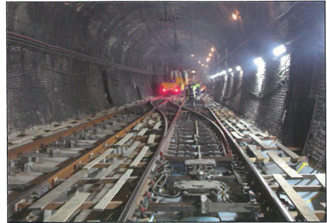
Fig. 7: Final preparations before pouring the initial concrete layer
