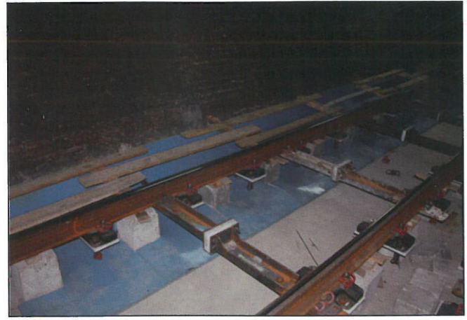
Fig. 6: Installation of the vibration isolating mats
