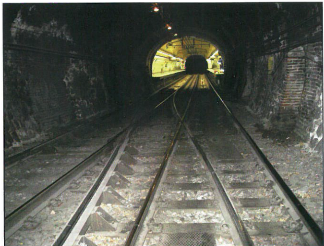
Fig. 1: A typical transition zone (ballasted turnout track) near a station
