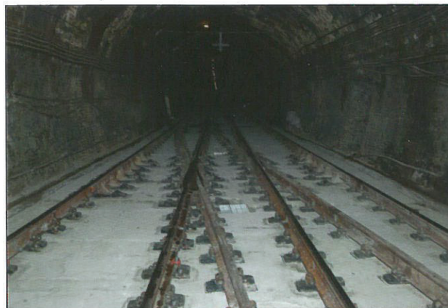
Fig. 10: Completed transition zone (turnout on a slab track mass-spring system)
