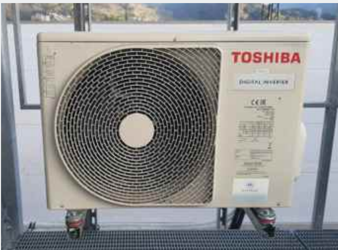
External air conditioning unit on wall bracket
