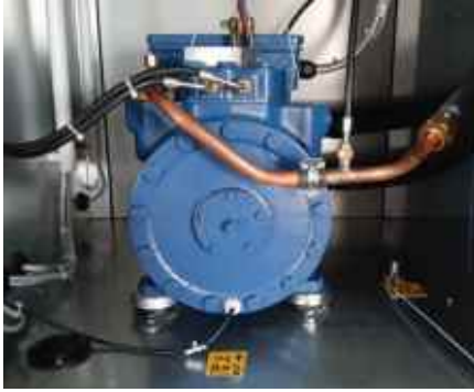
Rubber-metal bearing
