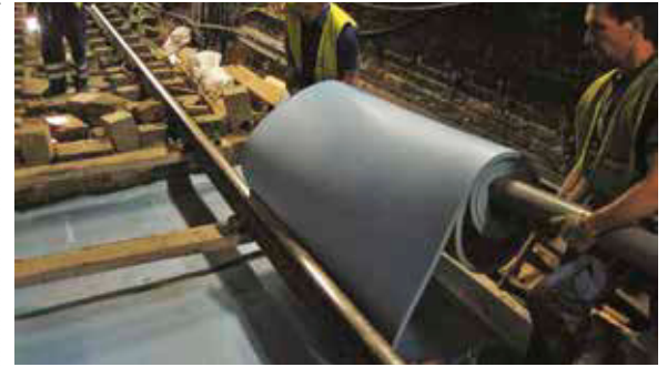
The vibration-suppressing mats bend easily and can be cut using conventional knives, making them simple to install.
