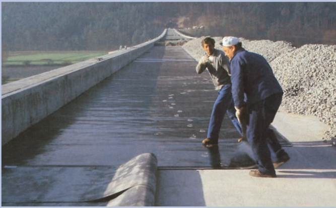
Fig. 2: Installation of the D 220 ballast mat on the Bartelsgraben Bridge in 1987
