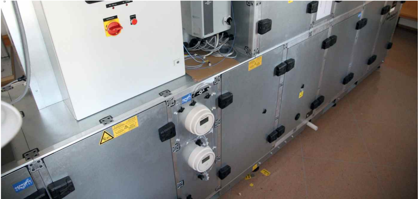
Complete unit with measuring points on the floor
