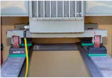
Vibration decoupled bearing of a distribution transformer
